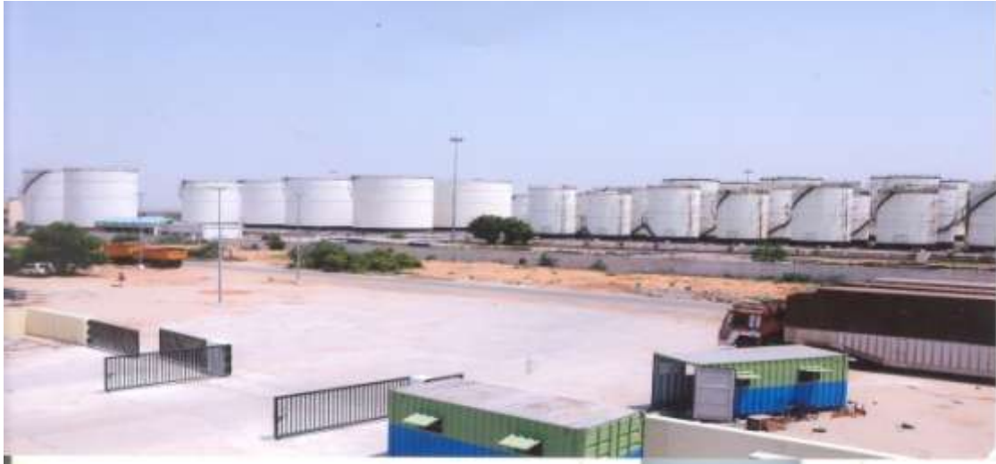
Fig. 4 - View of Tank Terminal
