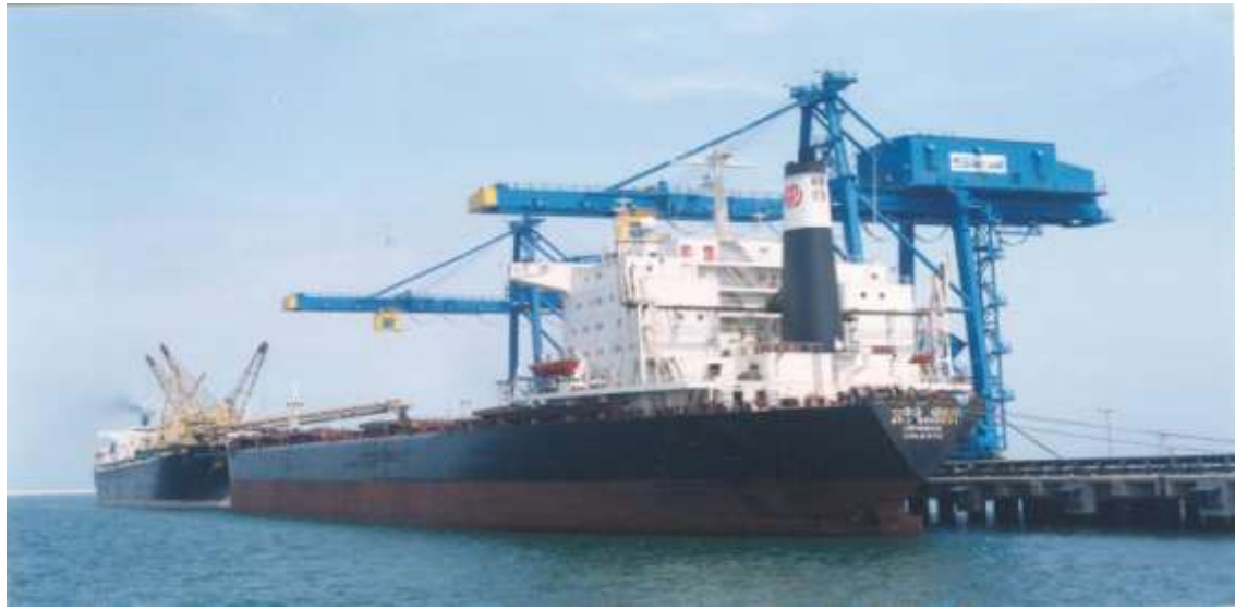
Fig. 2 - Coal berths Dedicated to TNEB
