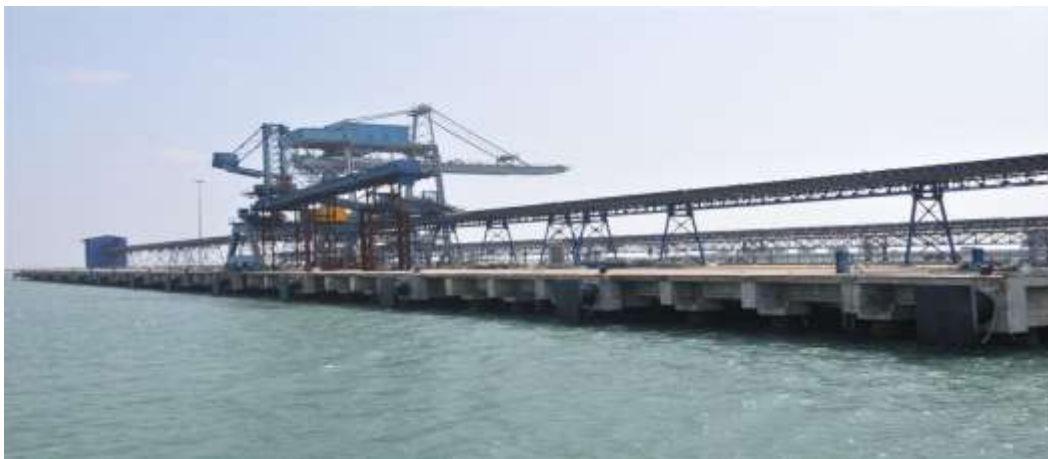
Fig. 6 - Iron Ore Jetty, ship loader and Conveyor System
